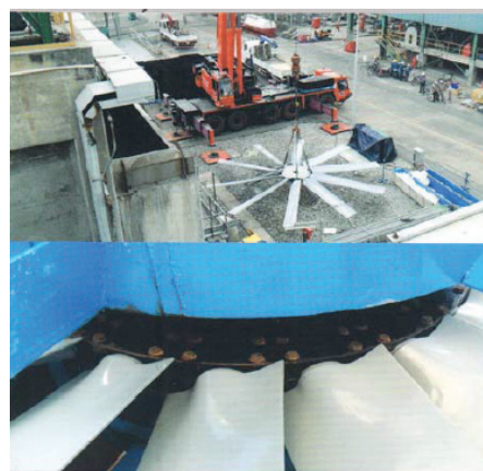
Figure 32: FRP Cooling Tower Fan
